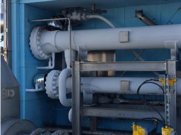
Figure 6: heat exchangers. LiN is guided past the cryogenic liquid to cool it down towards a sub-cooled state.
