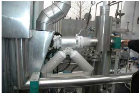
Flowmeter on-site (bend – no straight pipe before flow meters)
