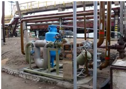
Flowmeter on-site (bend – no straight pipe before flow meters)
